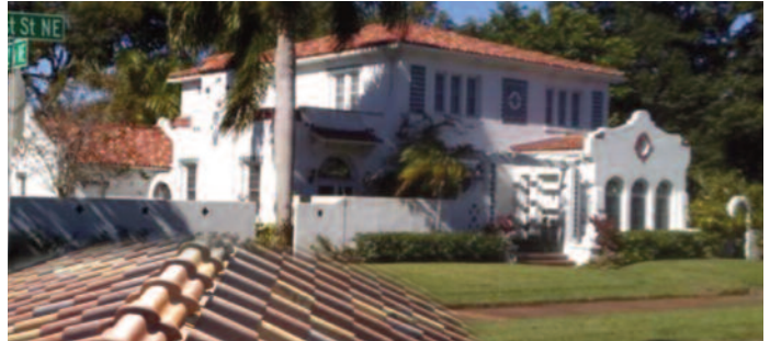
Vinoy Mansion (~75 yr Building- “Historic Property”)
