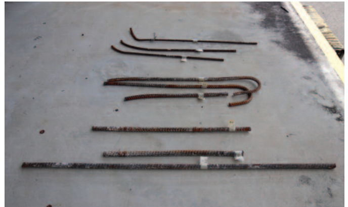
Samples of rebar recovered from the collapsed FIU pedestrian bridge, await transport to the Federal Highway Administration's Turner-Fairbanks Highway Research Center, where the samples underwent materials testing as part of the NTSB's ongoing investigation of the March 15, 2018, fatal, bridge collapse. (NTSB photo by Adrienne Lamm)
